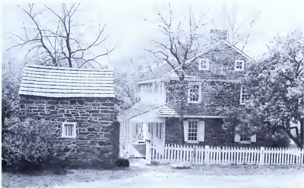
Daniel Boone's Homestead in Guilford, Pennsylvania. Built with the same brownstone siltstone
